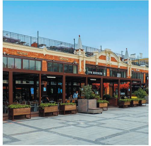
▼ DEPO OF THREE STATIONS, PHOTO: MOS.RU
